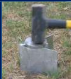
Driving post lock into ground
