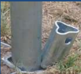
Inserting post and wedge
