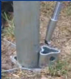
Inserting wedge removal tool
